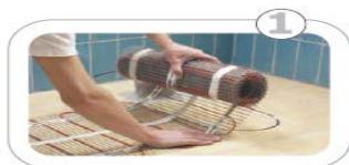
Roll the mat onto the floor
