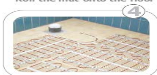
Ready to install tiles
